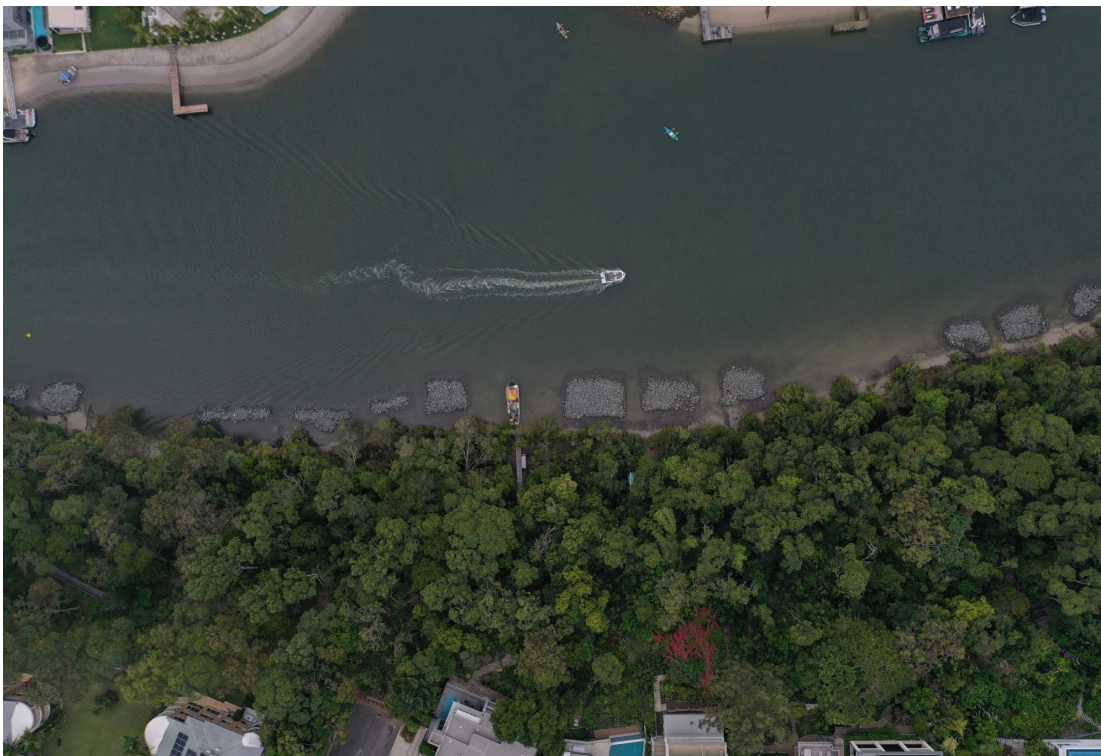
Figure 3 Aerial image of new constructed intertidal Sydney Rock Oyster Reefs in Noosa Estuary
